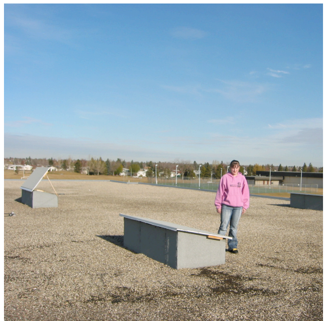
Figure 2. Typical Array of Detector Boxes on School Roofs
